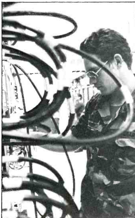
Mark DeWoody makes an adjustment to a Spectrum Analyzer, at The East Coast Telecommunications Center. The Center has a key role in the Space Shuttle program.
